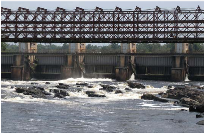
Hydroelectric plant, Democratic Republic of the Congo. Photo credit: UNEP.
